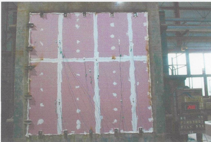
Unexposed face of the specimen after fire test
